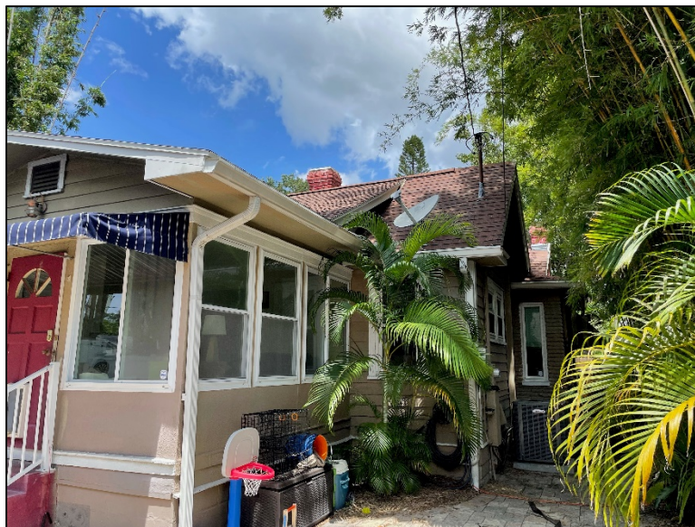
Figure 4: Rear and east side elevations of subject property, showing location of proposed addition
