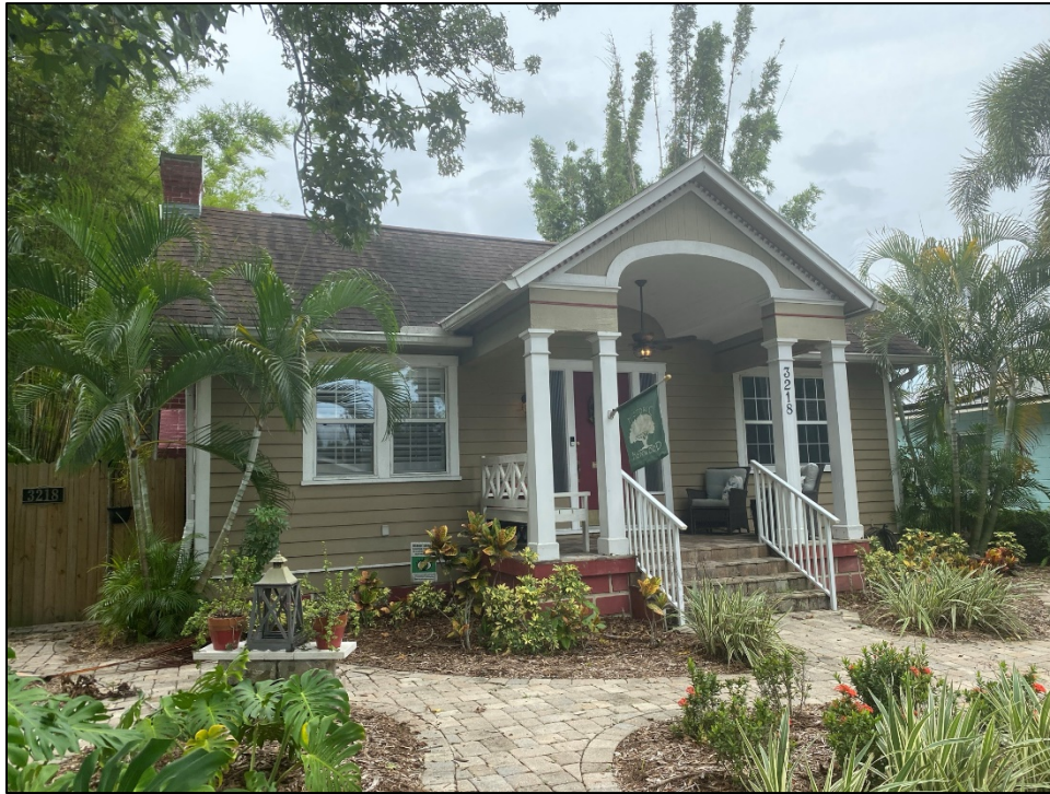
Figure 1: Subject property from 8 th Ave. N.
